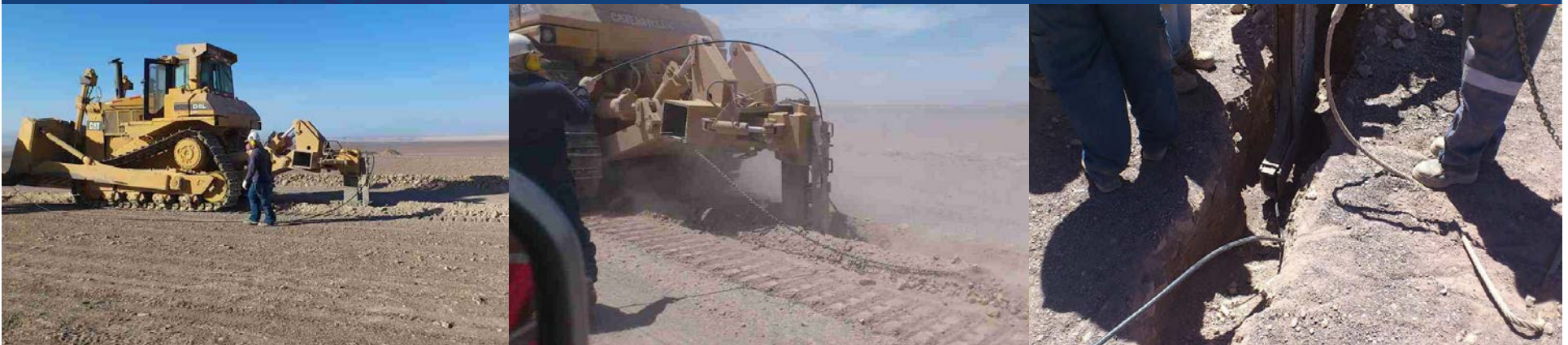
caterpillar equipped with “ripper” to insert the cable into the loose soil in the trench
