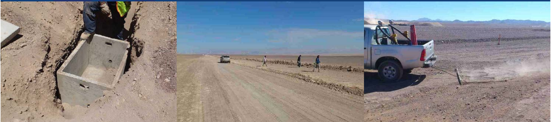
Installation of chamber (~every 4km), clearing and conditioning of the surface
