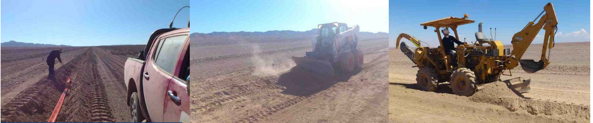
Warning strip and trench filling
