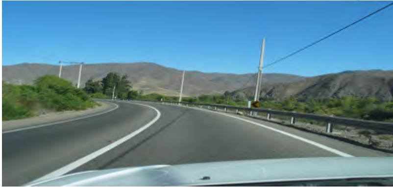
Typical public highway posts to La Serena. SLA with MTTR=4-6hrs
